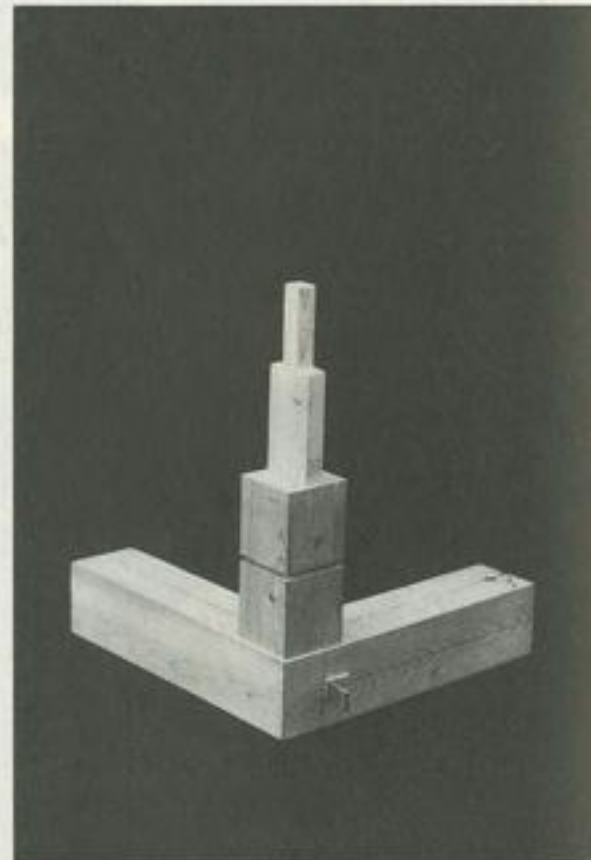
④ A column is set on top of the sill.
