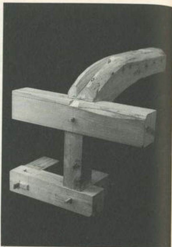
② The rainbow beam connects on the girder through the kabuto dovetail system.
