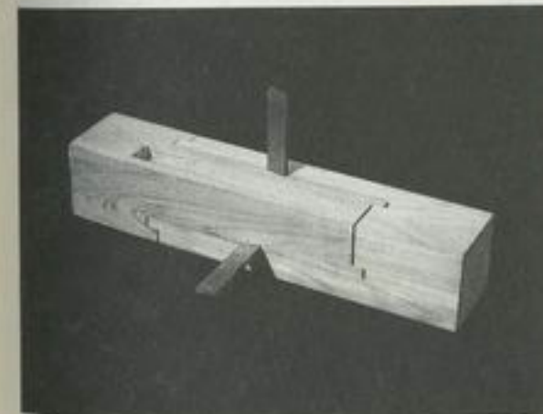
④ The splice is completed by inserting two keys.
